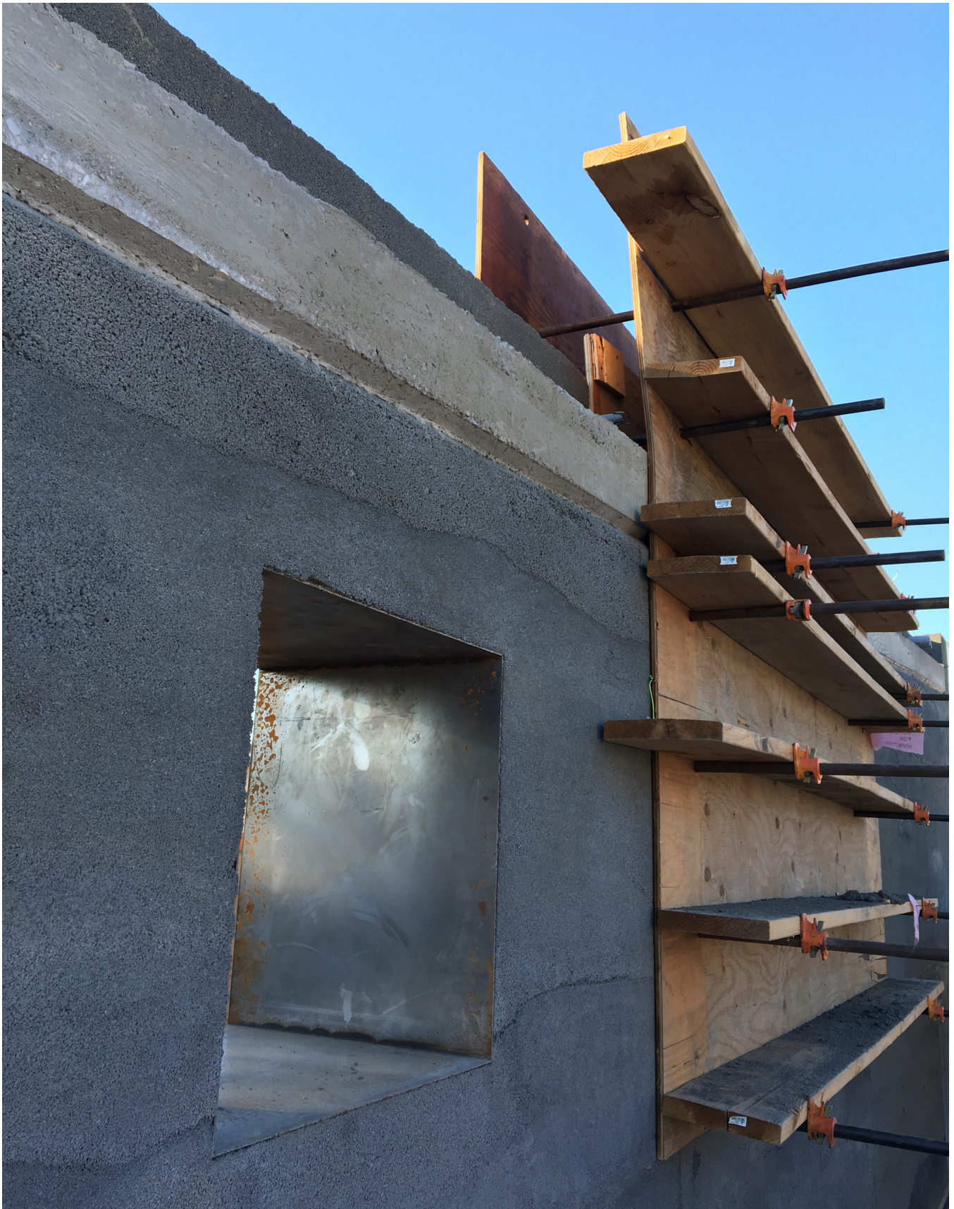
Figure 4. Wall and window forms, bond beam. Photo by Queston Kwolek.
