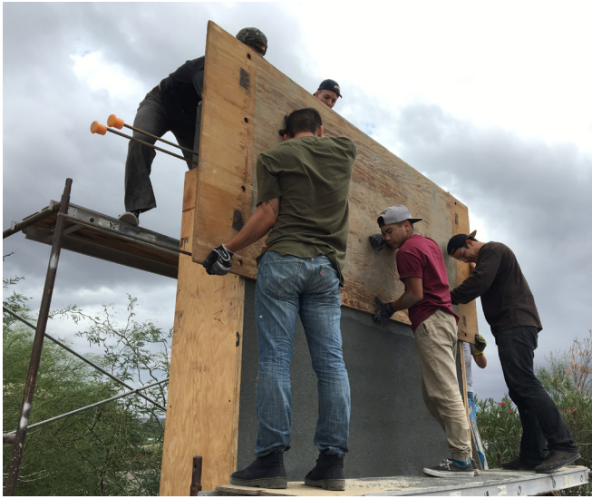
Figure 2. Plywood forms for scoria walls. Photo by Queston Kwolek.
